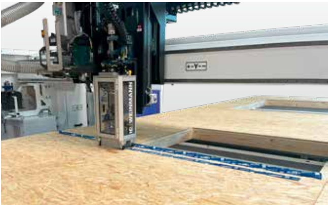
Application of sealing tape with the RAPICMASTER The innovative applicator, which was developed jointly by WEINMANN and pro clima, enables the automated, fast and precise application of sealing tape to the wall panel.
