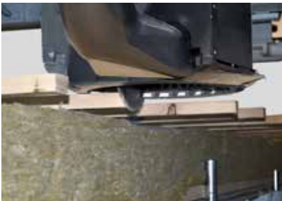
Formatting the roof battens
