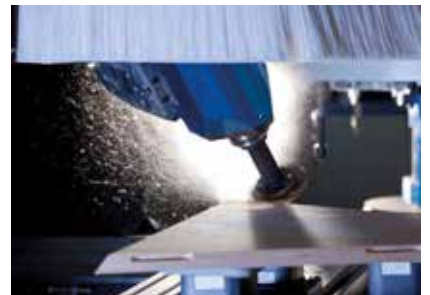
Trimming of angled grooves for panel connection
